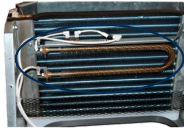
Plug in heat strip and controls, no miscellaneous wiring
